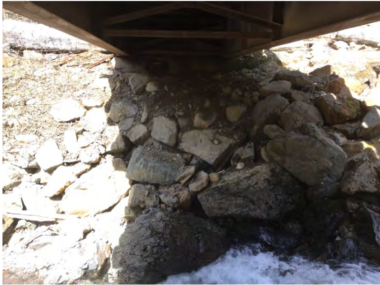
Right Bank Abutment when facing downstream
