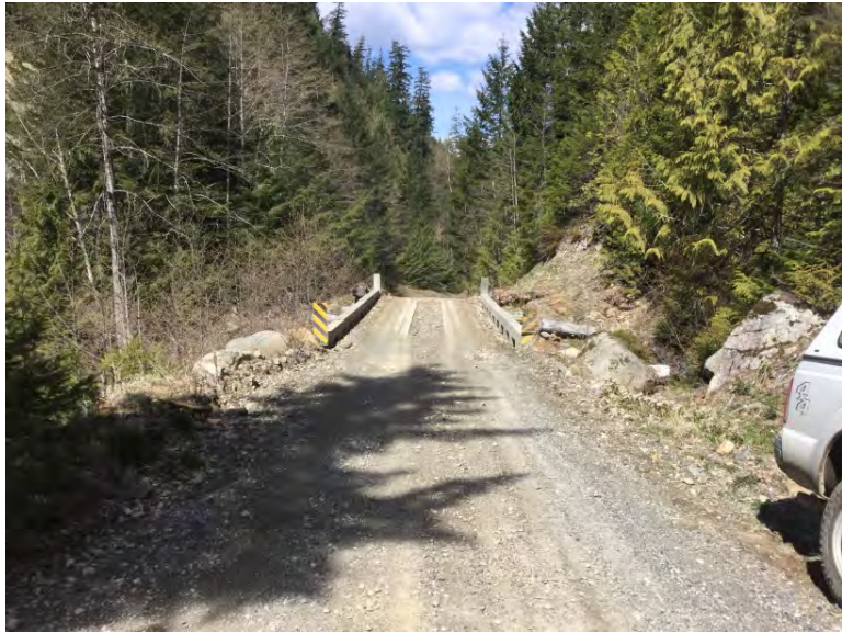
Approach from Left Bank when facing downstream
