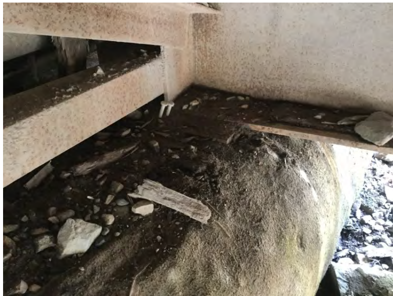
Upstream right bank bearing
