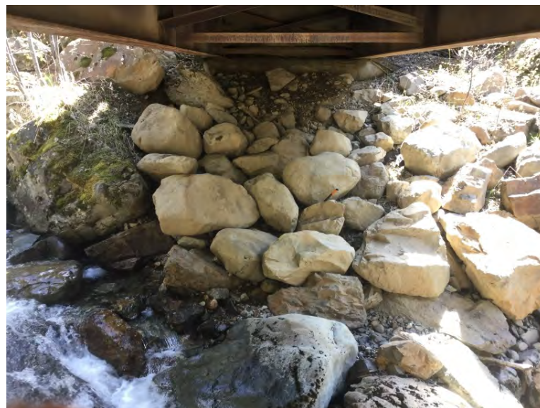
Left Bank Abutment when facing downstream
